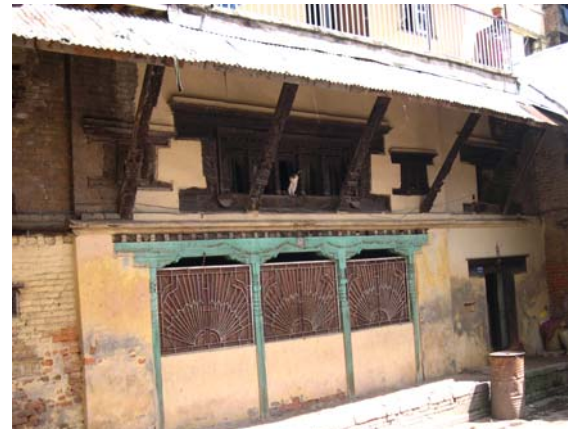
Plate 12: Closed dalan, additional roof and old elements
