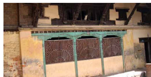
Plate 26: dalan with iron grill and partition wall to accommodate living space
