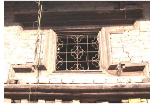
Plate 21: wooden lattice replaced by metal grill
