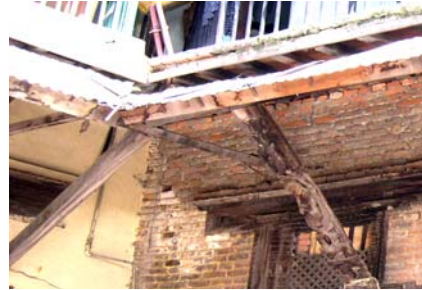
Plate 19: Missing strut replaced by ordinary timber
