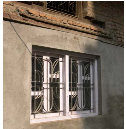
Plate 22: addition of new openings
