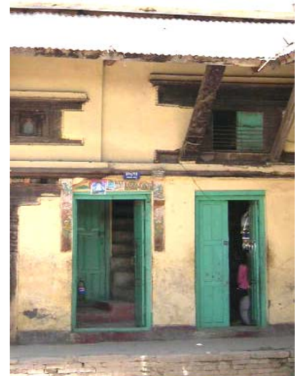
Plate 23: Addition of new openings
