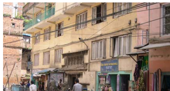
Plate 10: North wing showing facade
