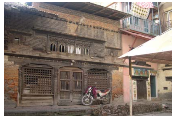
Plate 17: Multi level roofing
